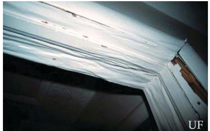
Figure 8. Blistered wood surface damage caused by the Formosan subterranean termite, Coptotermes formosanus Shiraki. Credits: Nan-Yao Su, UF/IFAS
