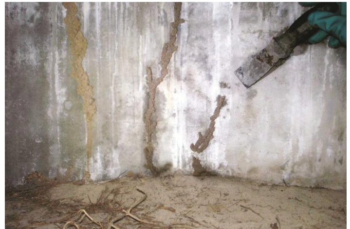
Figure 6. Mud tubes connect the colony in soil with wood in structure.
